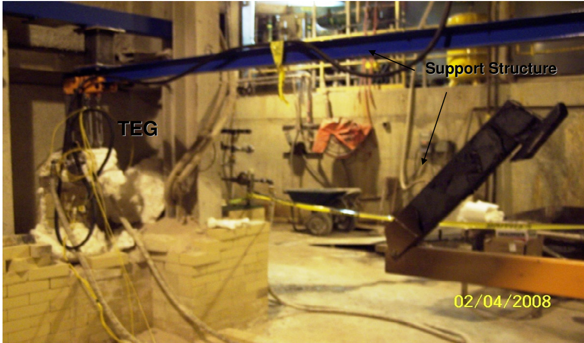
Figure 45 Photograph of in-plant test site, showing overhead support bar (blue) and the support used to minimize stress to the heat pipe during installation (folded back, orange) by supporting the heat pipe from below.
